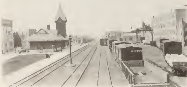
Kitchener Station and part of manufacturing district.
